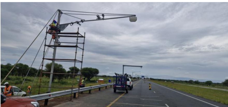
CAMEA's WIM system at WIMe pilot section in, South Africa.
