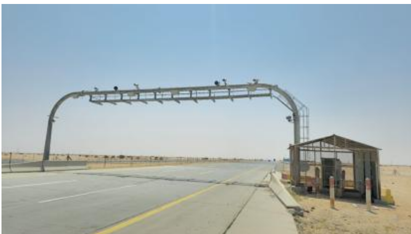
Pilot station in Saudi Arabia
