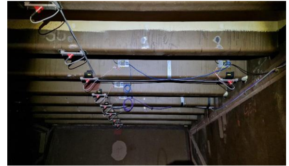
Steel structure bridge
