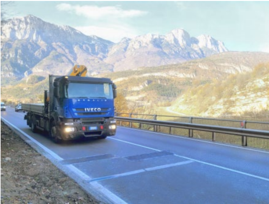
BISON LS Control System installed in Italy
