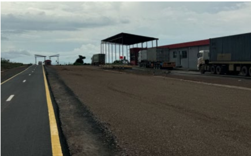
Integration of HS-WIM with a static weighbridge in South Sudan
