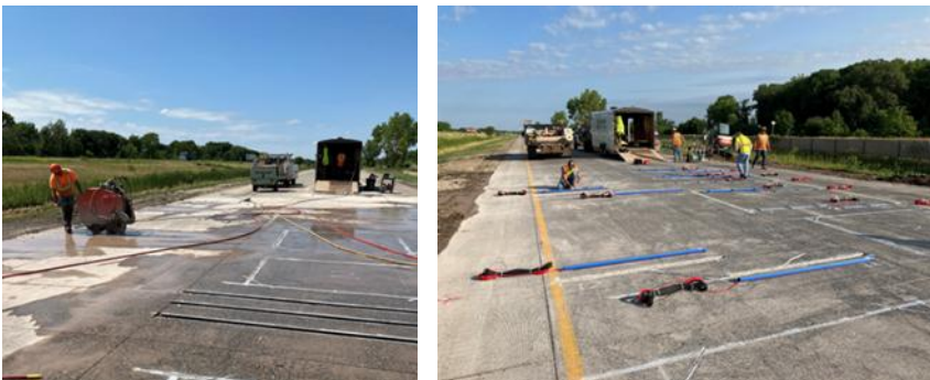
VectorSense and Quartz Sensor Installation
