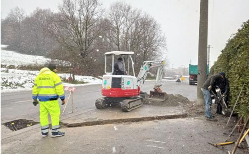
Installing a BISON WIM system during winter conditions.
