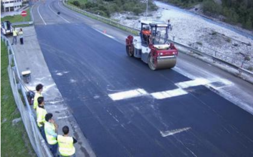
Resurfacing without removing the BISON bending plates.
