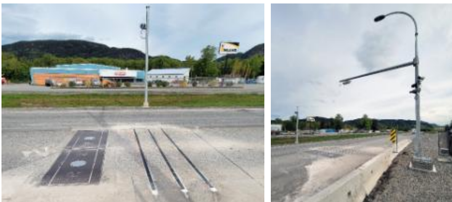
Terrace, BC Virtual Weigh Station – SLC WIM and TACS
