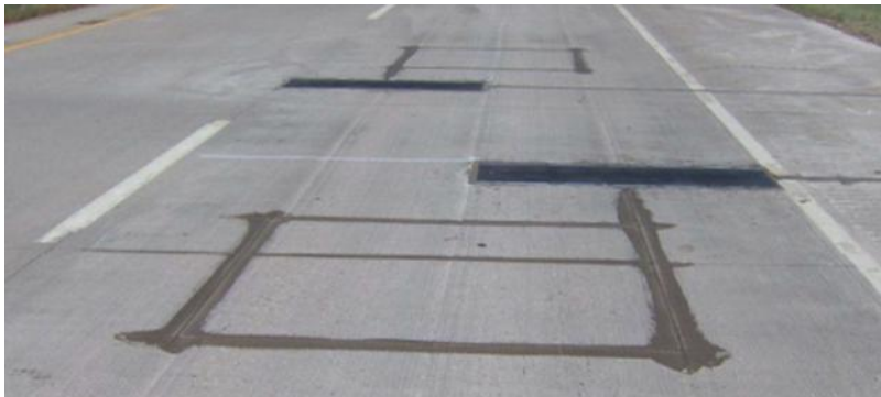
Original installation of WIM Scales and Loops.
