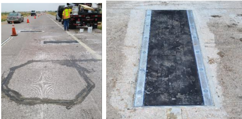
Site upgrade work at the WIM site and new Bending Plate
