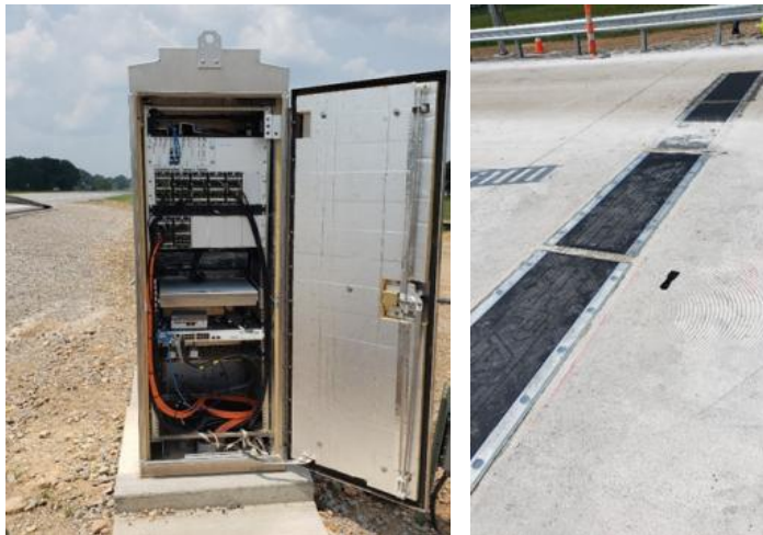
iSINC WIM Controller and IRD-PAT Bending Plate WIM Scales
