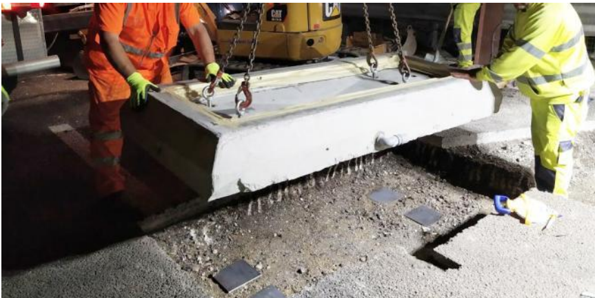
Installation directly in a reinforced prefabricated concrete.
