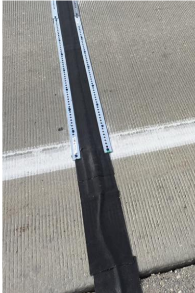
Portable WIM sensor installation
