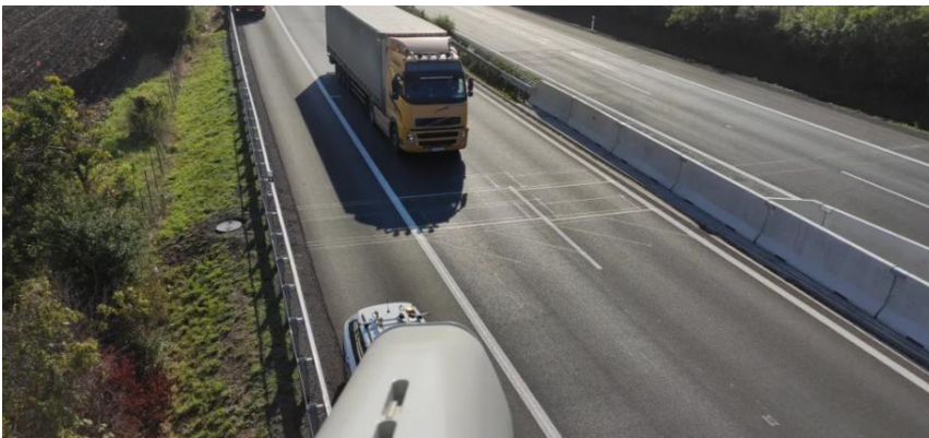
CrossWIM installed on a highway in Czech Republic
