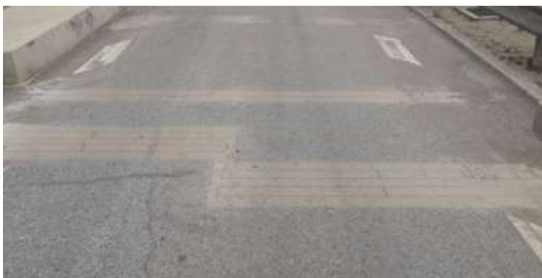
VanJee installed bar sensors into an asphalt road.
