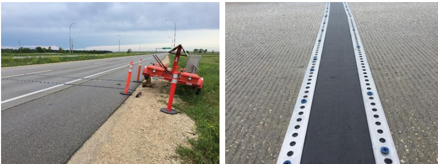
Installation of portable WIM system(left) and sensor (right)
