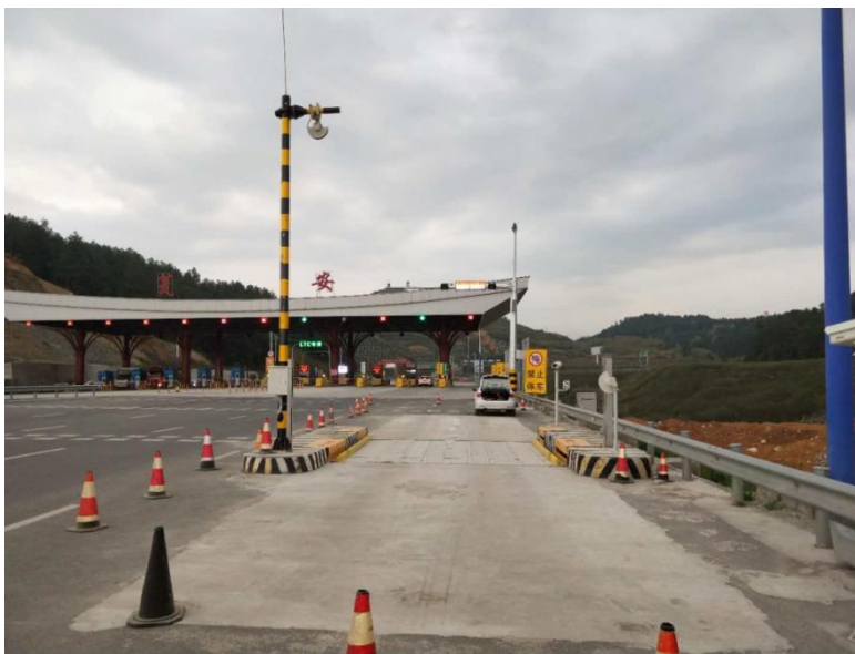
VanJee WIM system for 'No Entry' for overloaded trucks
