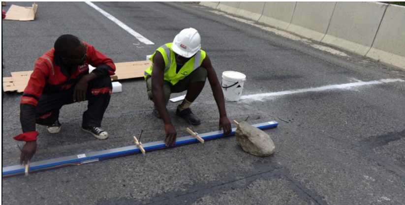
Installation of WIM sensors in Kenya.
