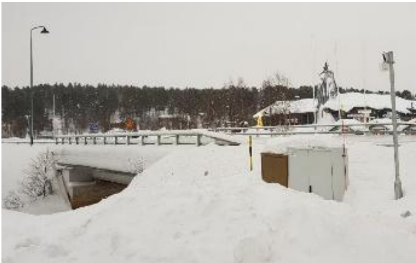
Bridge WIM system installed in Arctic Circle, Finnish Lapland
