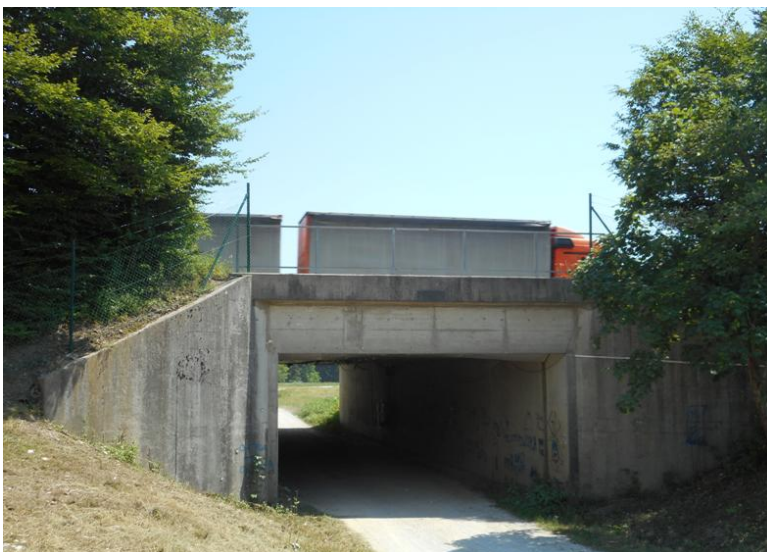
The studied bridge in Ljubljana, Slovenia
