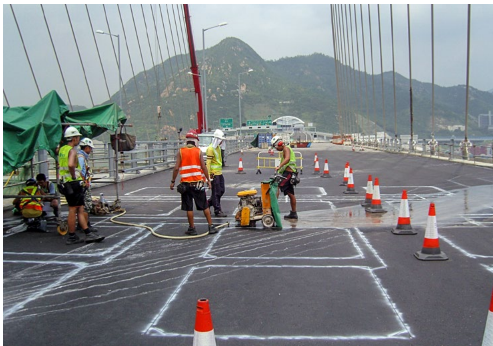
Figure 4.3: Example of a WIM system installed on a bridge in China
